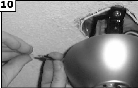
10 Make wire connections to power source using wire nuts provided. Make sure that no filaments are outside of the wirenut. After making the wire connections, the wires should be spread apart with the grounded conductor and the equipment-grounding conductor on one side of the outlet box and ungrounded conductor on the other side of the outlet box.
